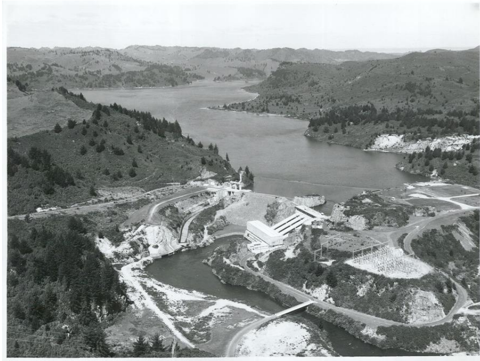
Figure 3 Aerial view of Ohakuri Power Station in 1969
