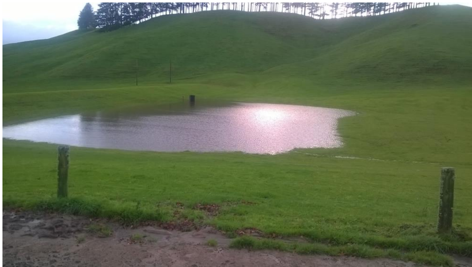
Example of a detention bund
